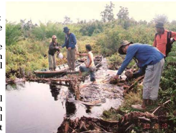
Repairing a dam
