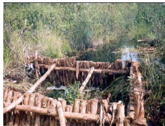
An example of dam construction
